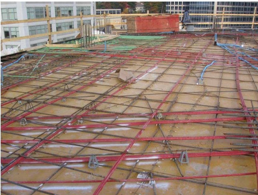
Unbonded tendons in the ninth floor slab of WPR.
